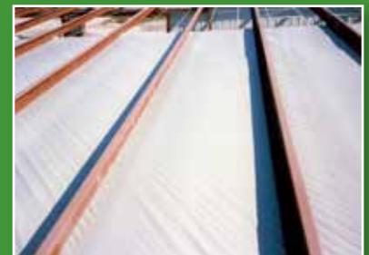
View of fabric liner positioned on strap platform and fastened to the structure.
