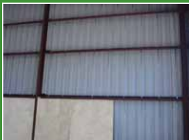
Secure the Fast-R™ insulation hangers to the wall structure with the punched arrows bent 90 degrees from the vertical.
