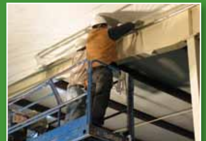
Fasten and seal the fabric liner edge to the rafter.
