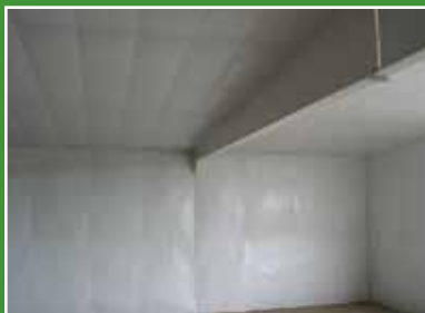
Fabric liner with steel straps installed to create clean, finished look.
