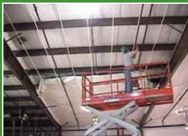
Install steel strap platform and the fabric liner across the bay.
