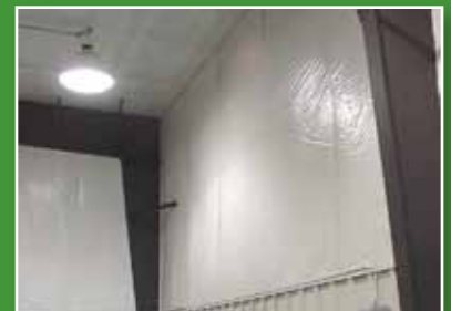
Finished wall and ceiling in manufacturing facility.
