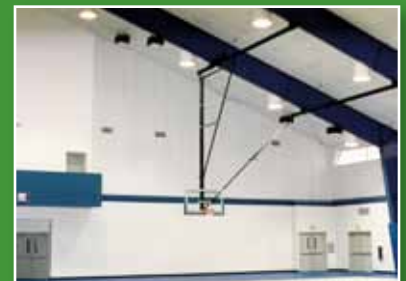
Finished ceiling and wall system in school gymnasium.
