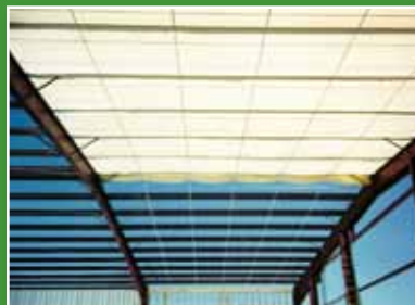
Large custom-sized fabric liner installs quickly on the steel strap platform.
