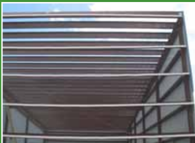
Quik-Stop™ thermal break tape applied to outside of girts.
